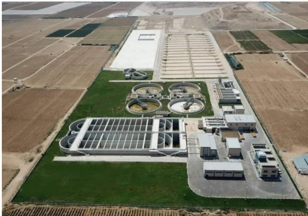
Figure 30: Wastewater Treatment Plant in eastern of Khan Younis Governorate
